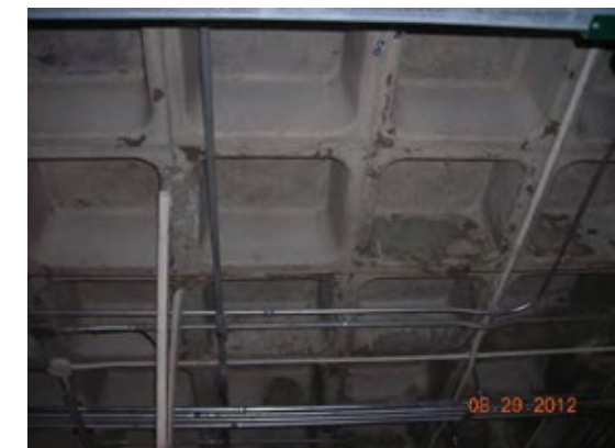
Photo 2 Waffle Slab Construction
