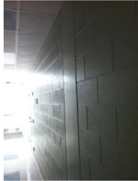
Photo 2 Concrete Block Infill Walls
