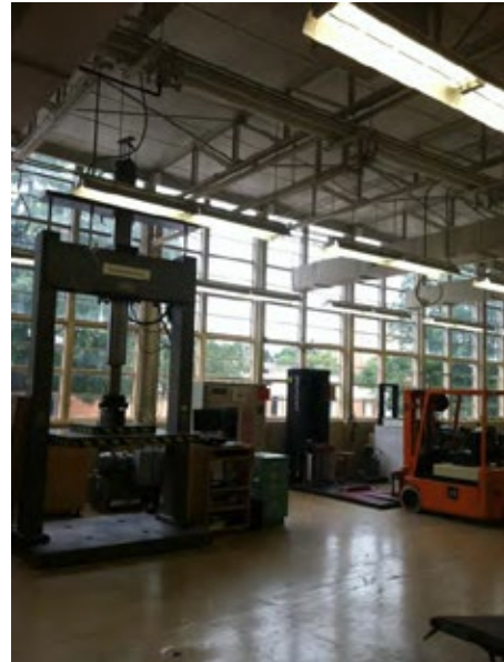
Photo 5 Asbestos Roof Form Deck
