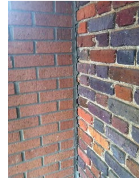
Photo 6 Stair Tower Addition
