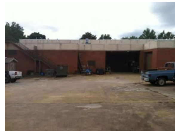
Photo 2 1974 Addition Rear Service Area
