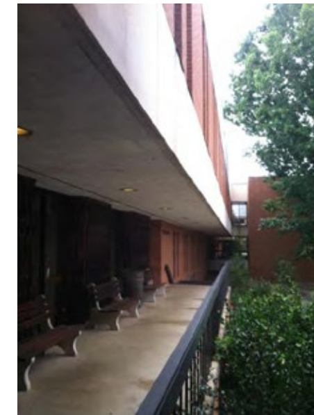
Photo 1 Cantilevered Second Floor
