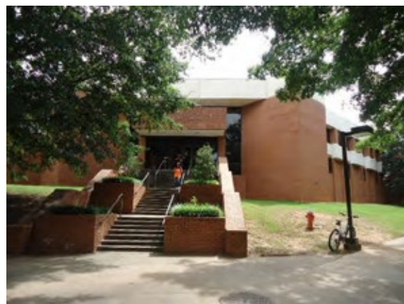
Photo 1 1974 Addition New Entry
