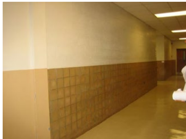
Photo 5 Interior Partition Walls
