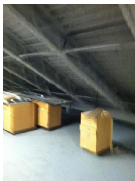
Photo 3 Lab Building Penthouse
