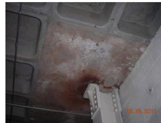
Photo 1 Column Support for Lift Slab
